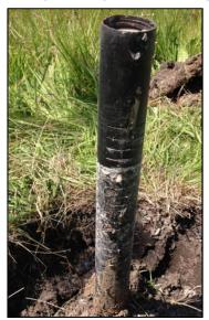
and reduce uncertainty. A monitoring well installation which has a slotted pipe from top to bottom (see figure) installed because the driller, "forgot to pick up lengths of plain pipe from the yard this morning," is unacceptable. What would be worse is if the 'monitoring well' was installed with plain pipe from top to bottom.
